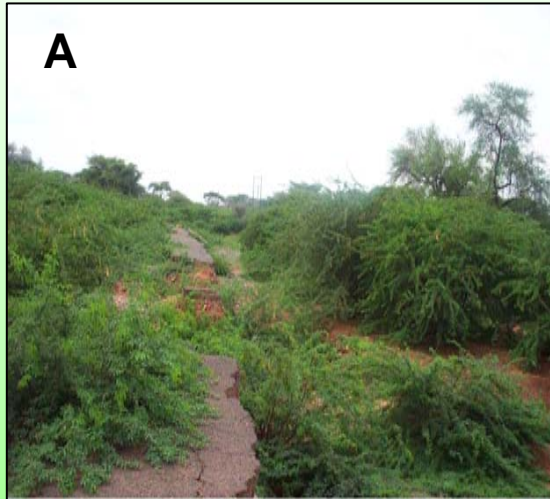
A. Over growing road network
